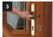
3. Install lever handle to the door using SES 3220 "Bolt Thru Screws".
