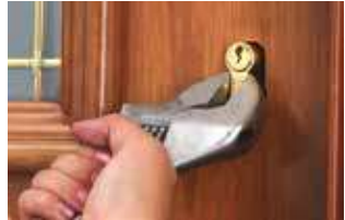
D. Tighten up with a switch wrench and swing it. (cylinder is exposed by at least 10mm).
