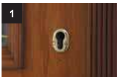
1. Install the security cylinder protector using "Bolt Thru Screws".
