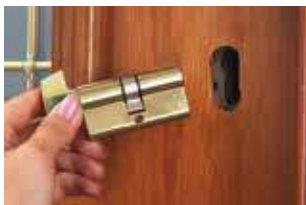
D. Put in a new profile cylinder.
